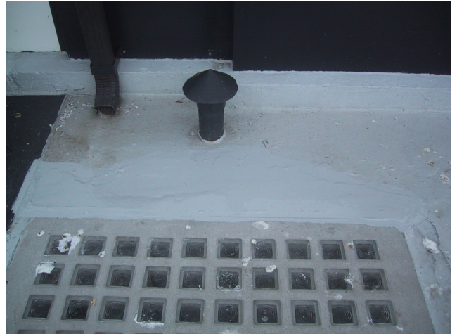
A ventilation pipe on the deck of the Light.
