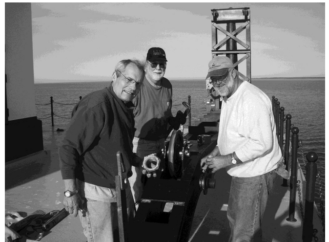
Don Gries, Ken Walker, Meade Gable assembling the crane's boom, August 2, 2008.
